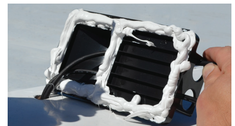
Underside channels guide adhesive dispensing around screws, drilled hole and plate perimeter
