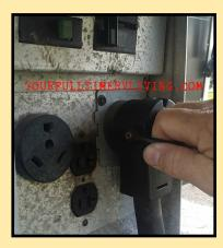
If every 120-volt appliance is turned off in the RV, this is not such a big deal. But that is usually not the case. Plugging and unplugging from the electrical pedestal with electrical load can create an arcing condition. This could damage whatever was turned on inside the RV! Over time, continued repetition of this action can lead to plug damage.
